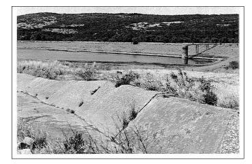
Google Earth images of the reservoir taken in 2004, 2011, 2013, 2015, 2018, 2021 show the reservoir full or part full. Empty in 2022 and February 2024. The diversion dam and inlet channels can still be seen clearly on the Google Earth images, although the part of the inlet channel shown in the photo suggests considerable renovation might be required.
